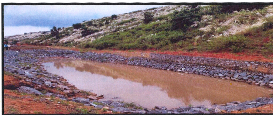
Siltation Pond for Treatment of Mine Seepage Before Discharging into Surface Water Bodies
