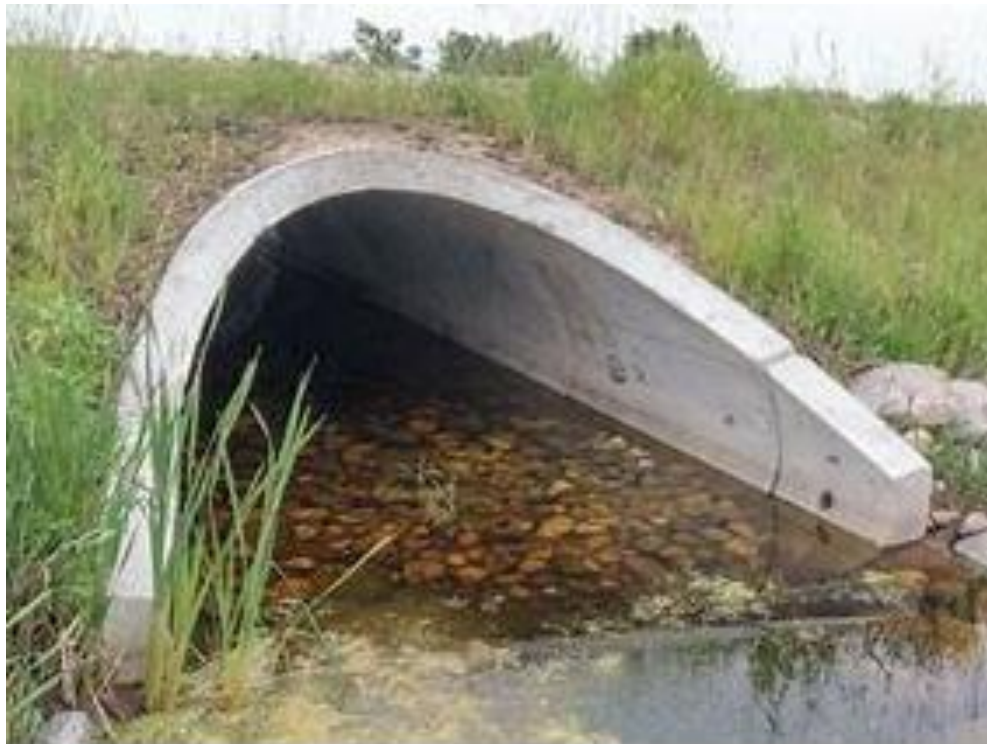
Figure- Design culvert structure of canal or water supply passing through wild life area
