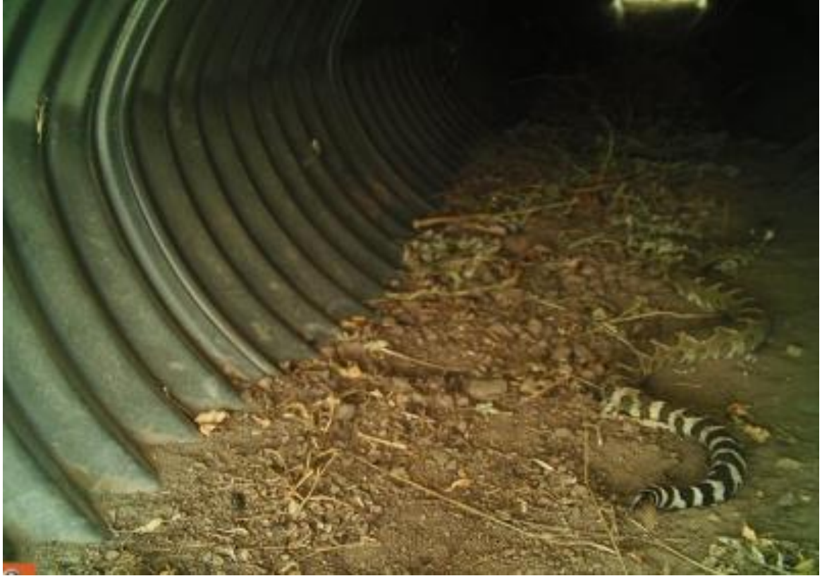
Fig: 5.7 A model tunnel for snakes, lizards and amphibian movement near highway.
