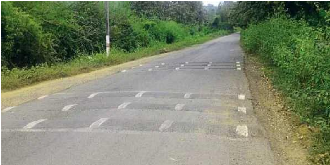
Fig. 5.5 Model speed breakers to be made during laying the road.
