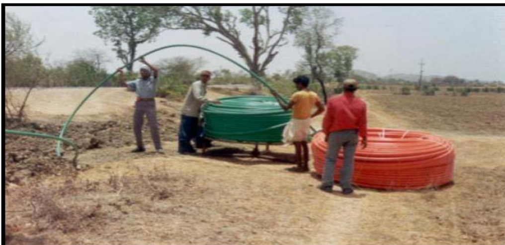
Using De-coilers at Site
