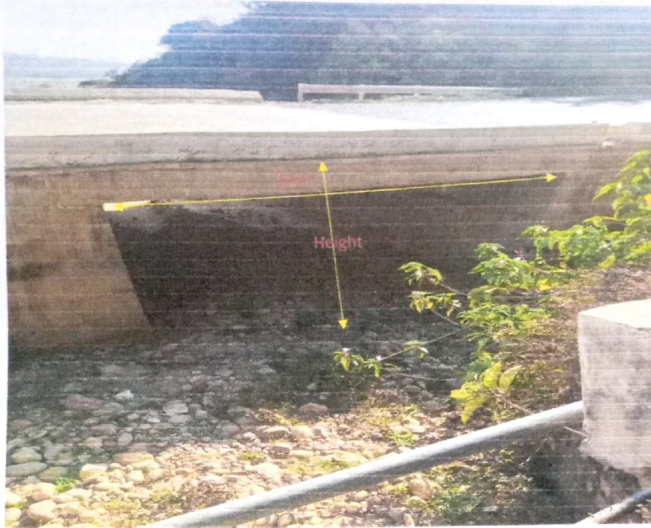
Fig.2 : Dimensions of an underpass determining its openness ratio
