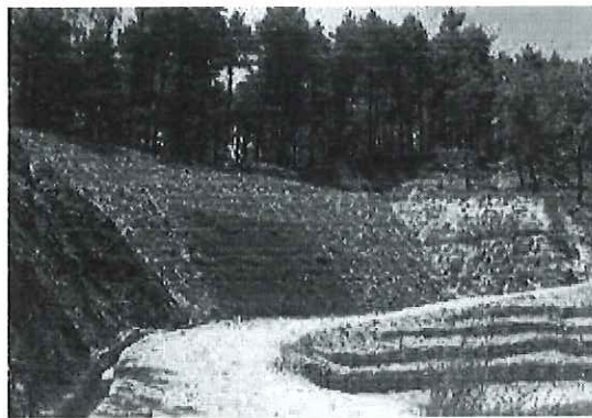
Slope Protection using Bio engineering techniques
