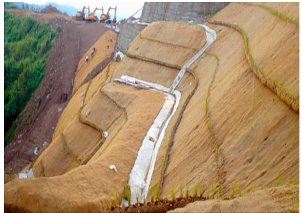
Use of Geo-mats for Slope Stabilization
