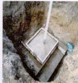
Stub Footing concrete
