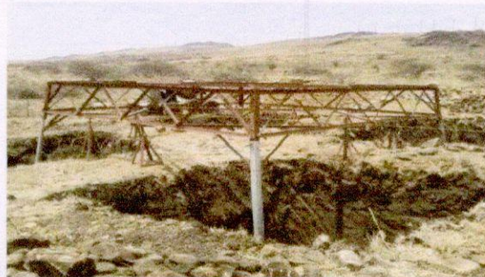
Stub setting & Template Assembly
