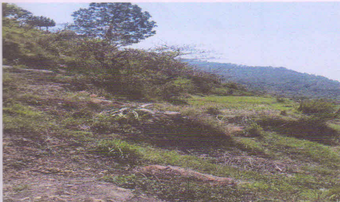
Dumping yard G(Chainge 4/38)
