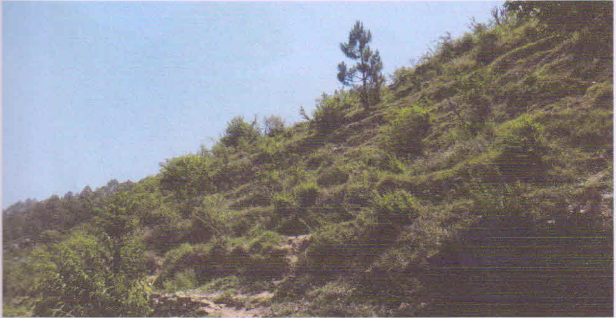
Dumping yard E(Chainge 2/20)
