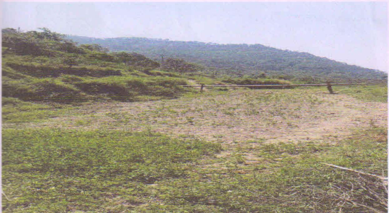
Dumping yard F(Chainge 3/35)
