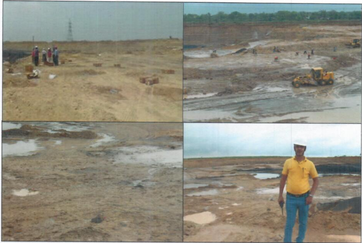
Photograph 2. View of the charging and connection with Nonel initiation device at North West face of Barjora (N) Coal Mine.
