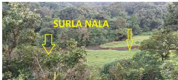
Figure 17: Downstream side View of Surla nala/diversion site
