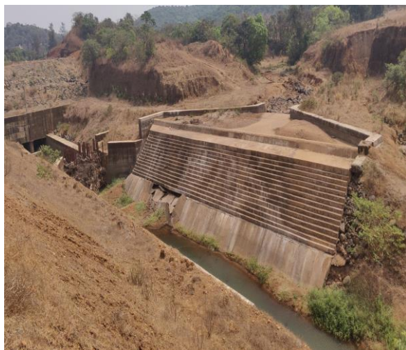
Figure 3: Existing Delivery chamber at project site
