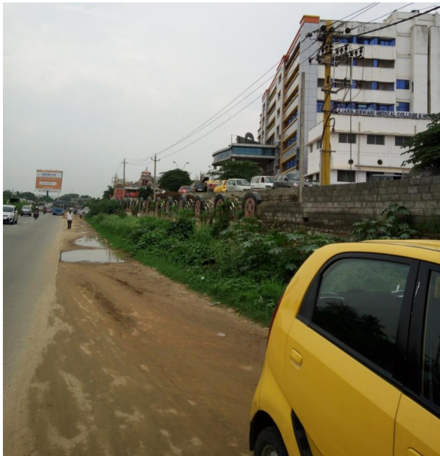
Alignment terminating on Mysore Road at Ch. 10+770 beside Rajarashwari Medical College & Hospital.
