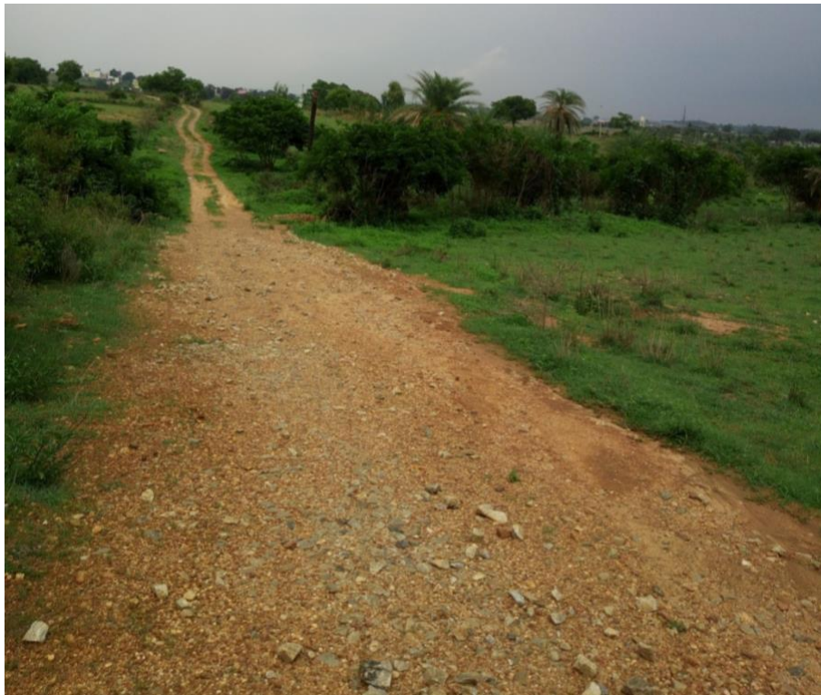
Alignment Crossing over existing kuccha road at Ch. 9+000.
