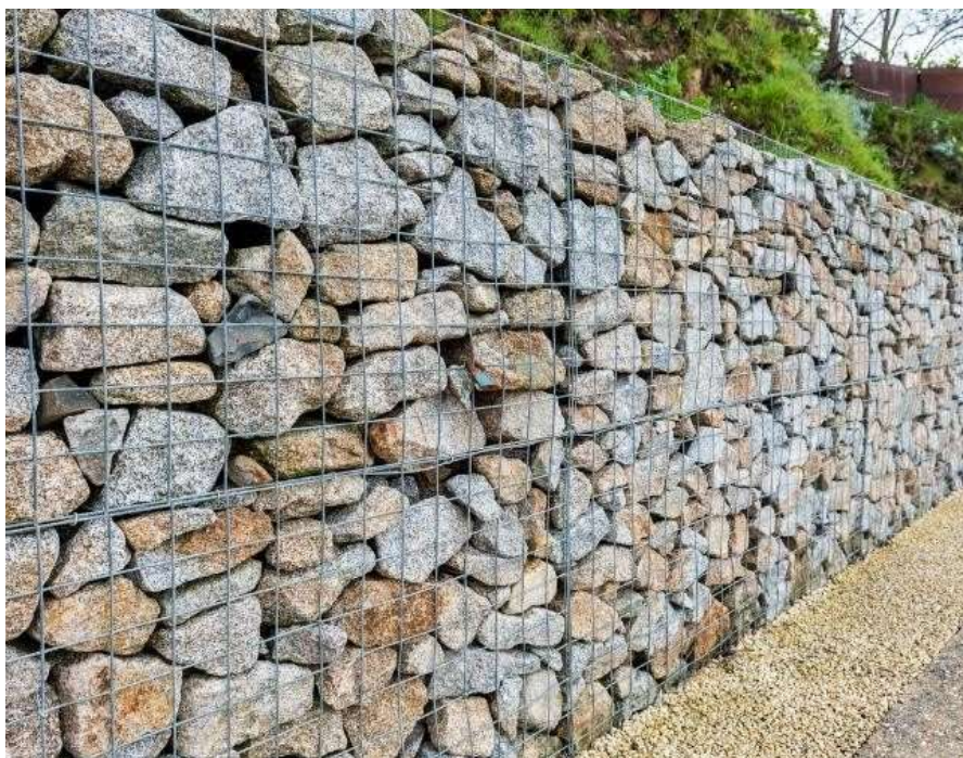
Figure 51 Typical Gabion Wall
