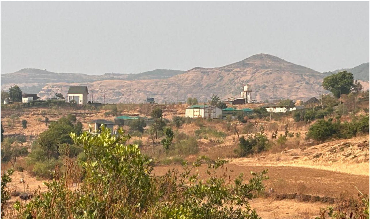
Figure 9: Housing structures in project site (> 600 m)
