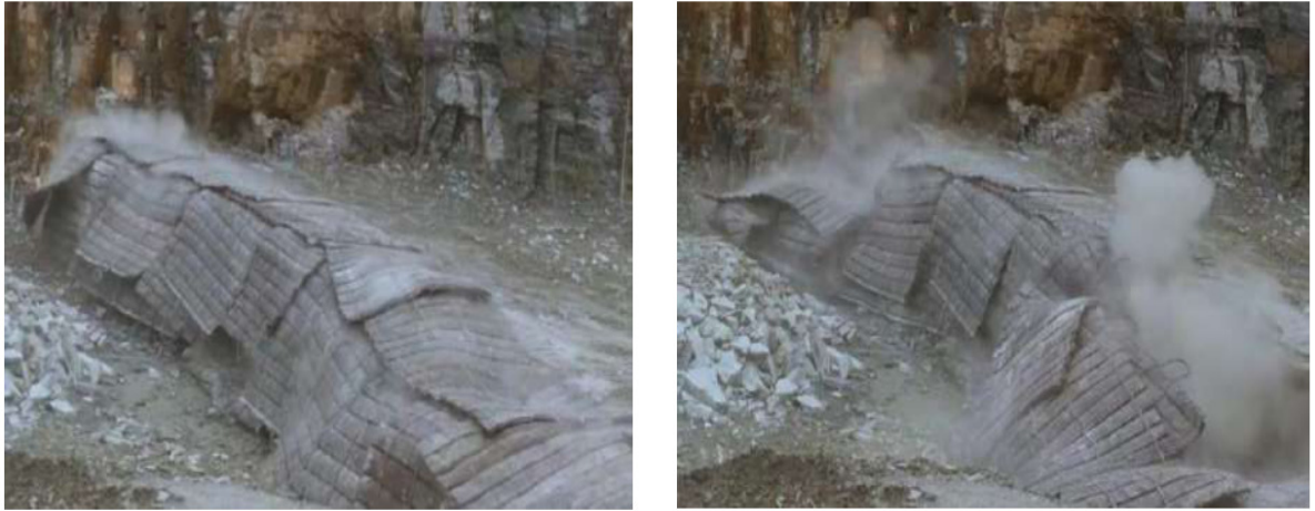
Figure 15: Photographs of blasting operation with blasting operation with blast mats
