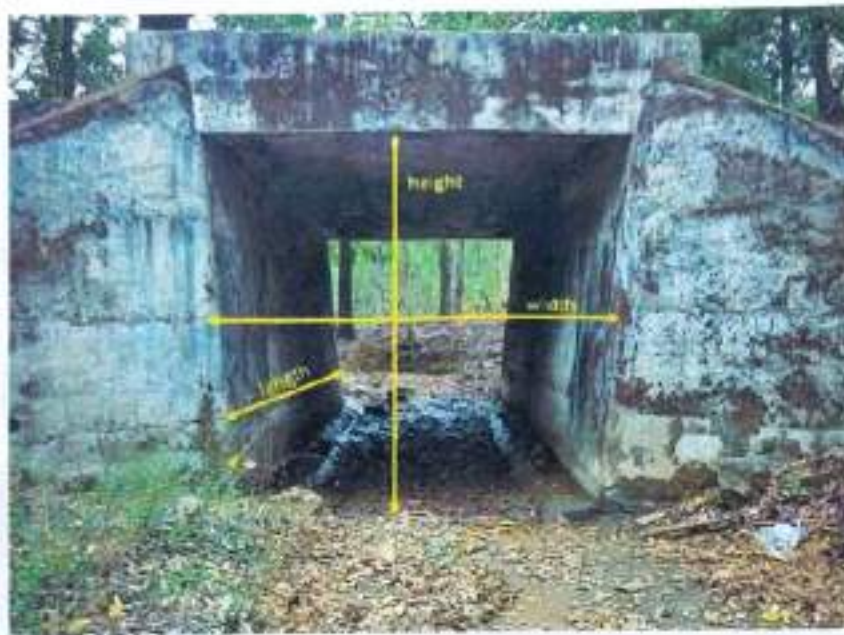
Fig.2 : Dimensions of an underpass determining its openness ratio
