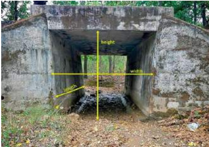
Fig.2 : Dimensions of an underpass determining its openness ratio
