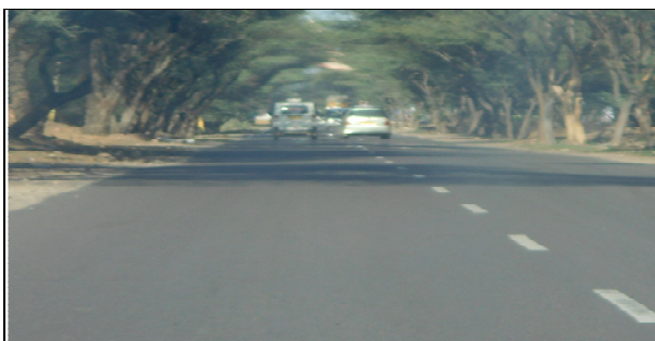
At Km. 165+000 to 166+000 Good Pavement Condition
