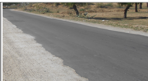
At Km. 203+000 to 205+000 Good Pavement Condition
